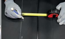
Fold back the top liner and mark the bottom sheet every  $\pm 10$  cm at 1 cm from the marked edge.
