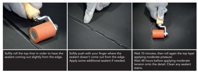
NOTE: one line of sealant is usually enough. For extra security, it is possible to add a second line of sealant at 50 mm from the membrane edge.
