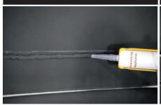
Clean the seaming area with a damp rag and apply a continuous line of sealant over the marks (1 cm from the edge) at a speed of  $\pm$  6s/10cm (min. 5 mm bead width) while the liner is still damp (not wet).
