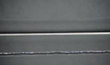
IMPORTANT: The line of sealant must be homogeneous. In case of thinning, apply additional sealant
