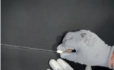
Mark the bottom sheet at the overlapping edge with a white marker.
