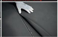
Reposition the top liner over the fresh sealant, respecting the marked edge.
